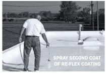
the second coat until the first coat has fully cured. Applying the second coat before the first coat has cured may result in slippage, crazing, or cracking of the coating.
