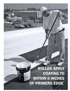
Allow the first coat of **RE-FLEX COATING** to cure before applying the second coat. Cure time is dependent upon ambient temperature and air moisture levels. Sunny days with moderate temperatures and low humidity will reduce cure time before the second coat can be applied (over-night to 24 hours). Overcast days with cool temperatures and higher moisture levels will prolong the cure time (24 to 48 hours).
