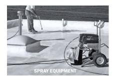
The first coat of Re-Flex Coating must be completely cured before any foot traffic is allowed. All equipment and other materials, foot traffic, etc. that make contact with the Re-Flex Coating must be clean and free of dirt, debris, and other contaminants.
