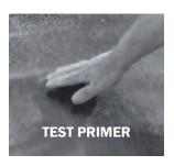
Before applying the first coat of **RE-FLEX COATING**, test the Primer for proper dryness by applying finger pressure. The finger should not slide over the Primer. The Coating Primer should be dry and tacky, not wet and stringy.
